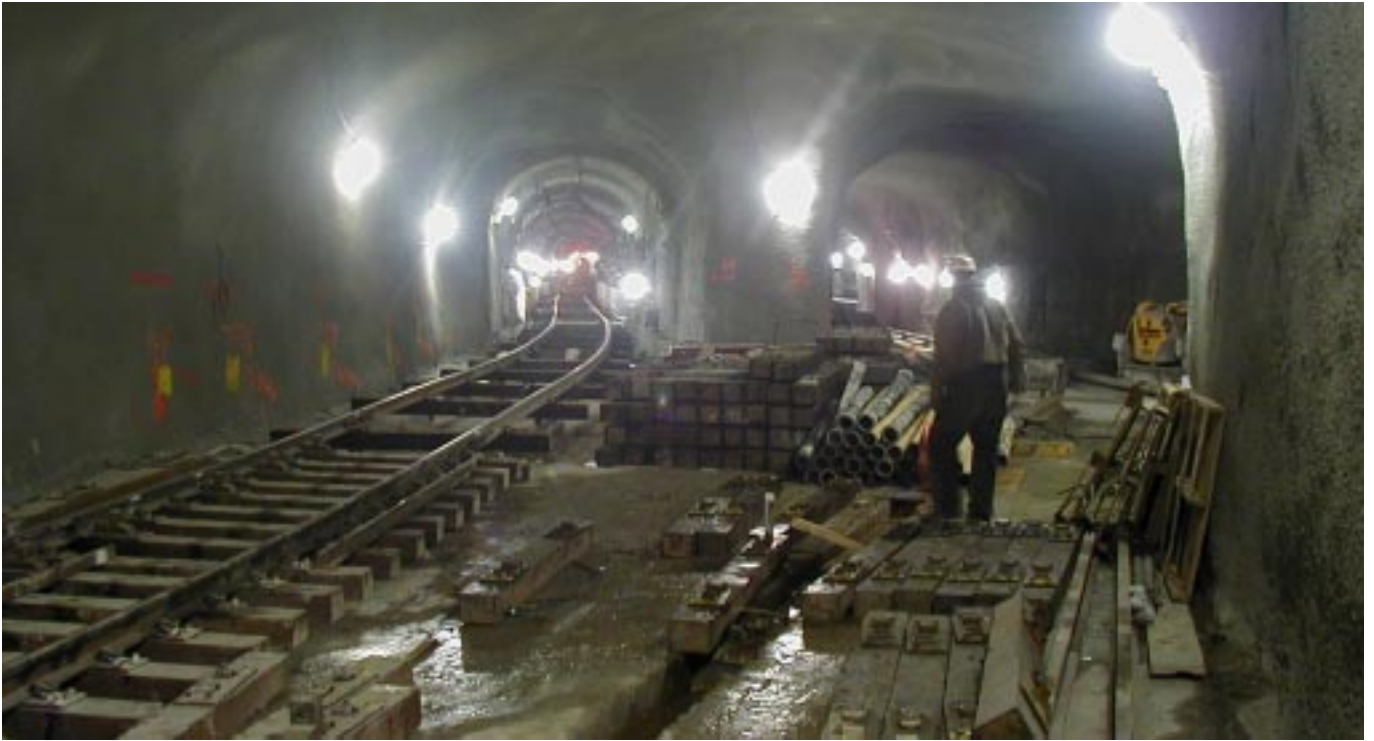
Everything in the tunnels had to be demolished and hauled out.
