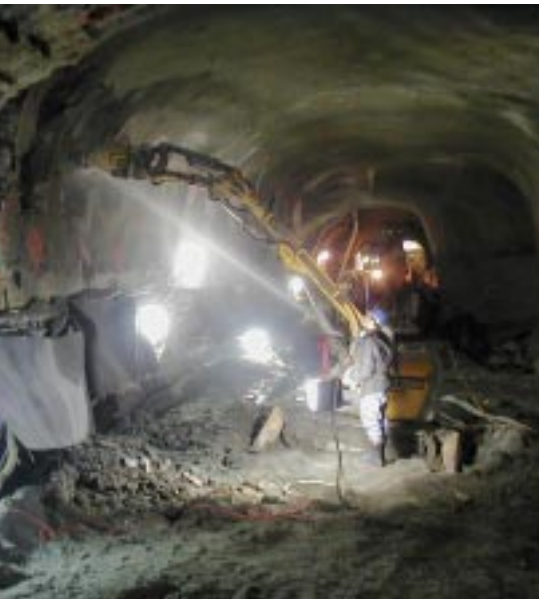
Brokk machines removed the concrete between the steel I-beams.
